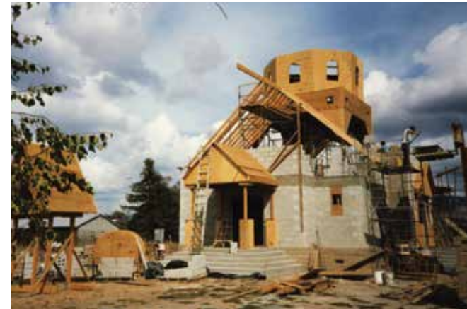
Church construction, September 1986
